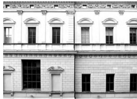
Fassadenansicht Altbau Facade view, old building
