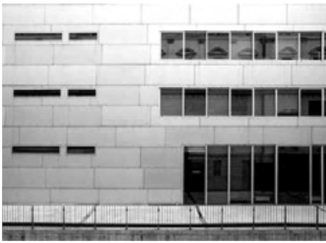
Fassadenansicht Neubau Facade view, new building
